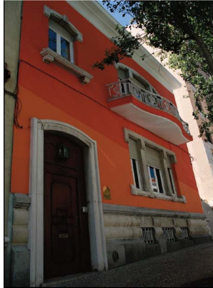
Headquarters, Rua Tomás Ribeiro, Lisboa
